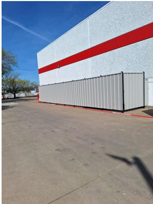
View of the outdoor storage area with the metal fence.
