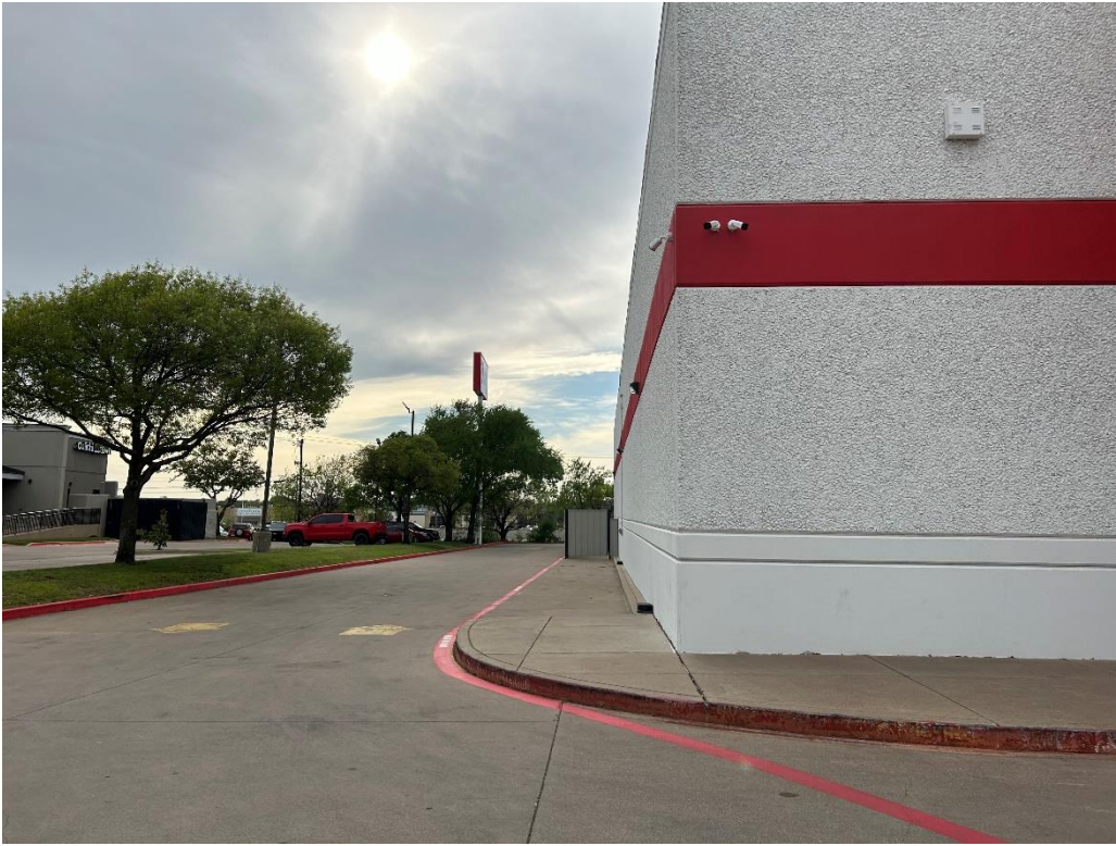
View of the outdoor storage area with metal fence
