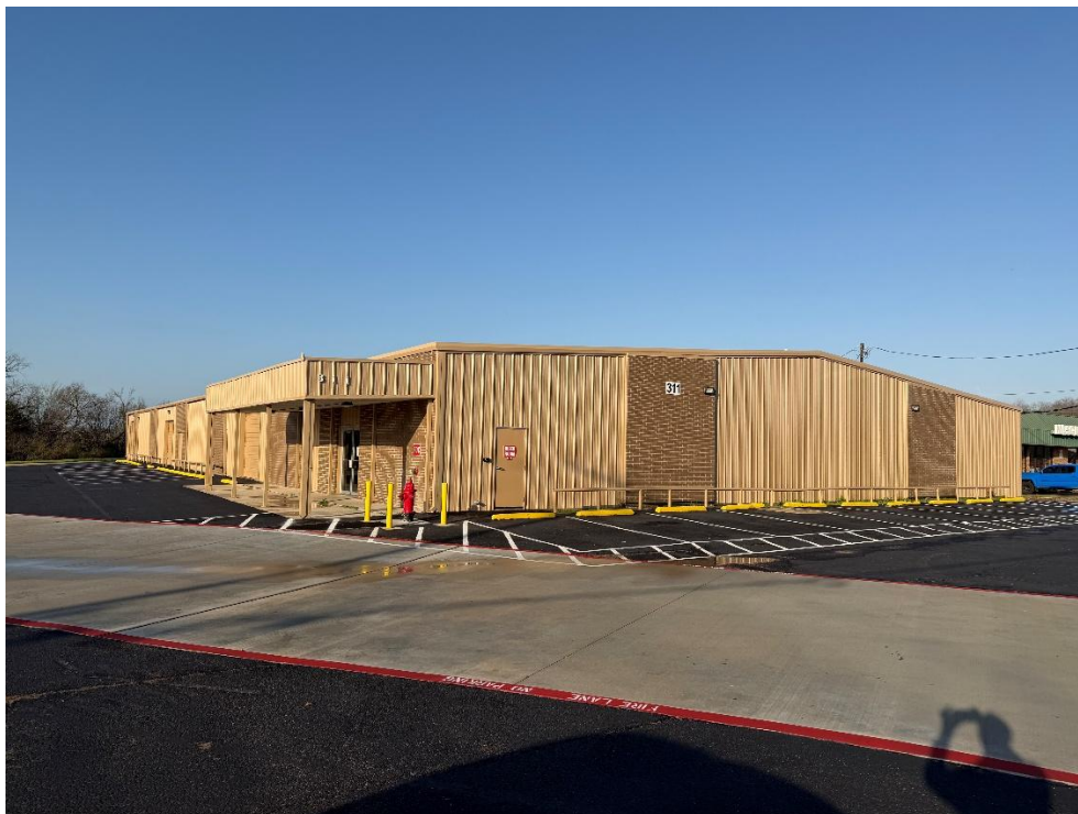
Former Skating Rink adjacent to the subject property
