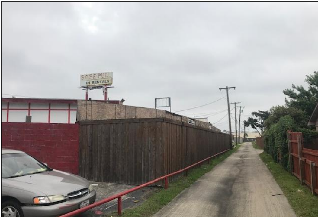
Rear view of the property showing screened area for storage.
