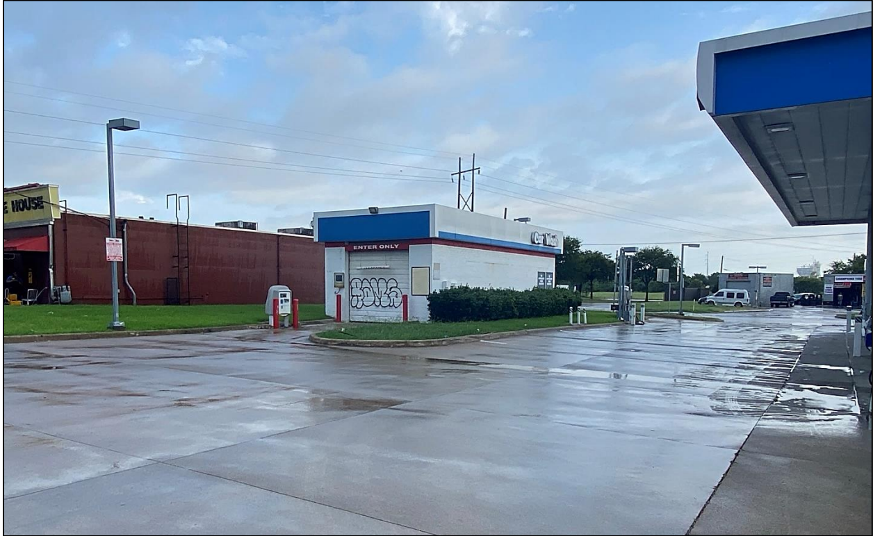
Existing tunnel carwash, facing northwest.
