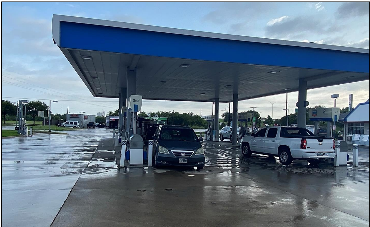
Existing canopy and fuel pumps, facing north.
