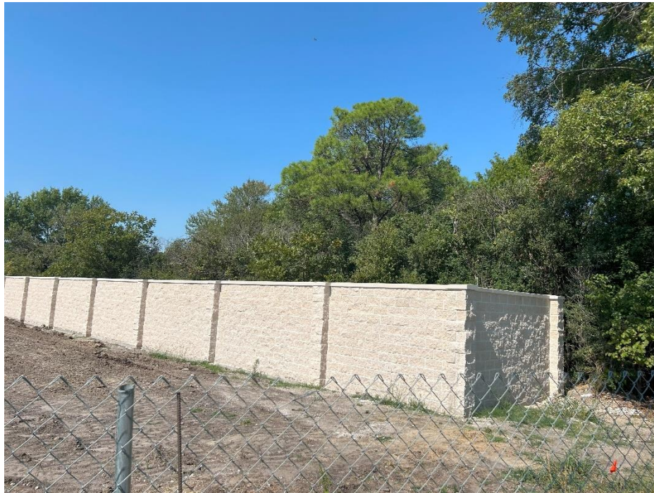
East end of the CMU Wall
