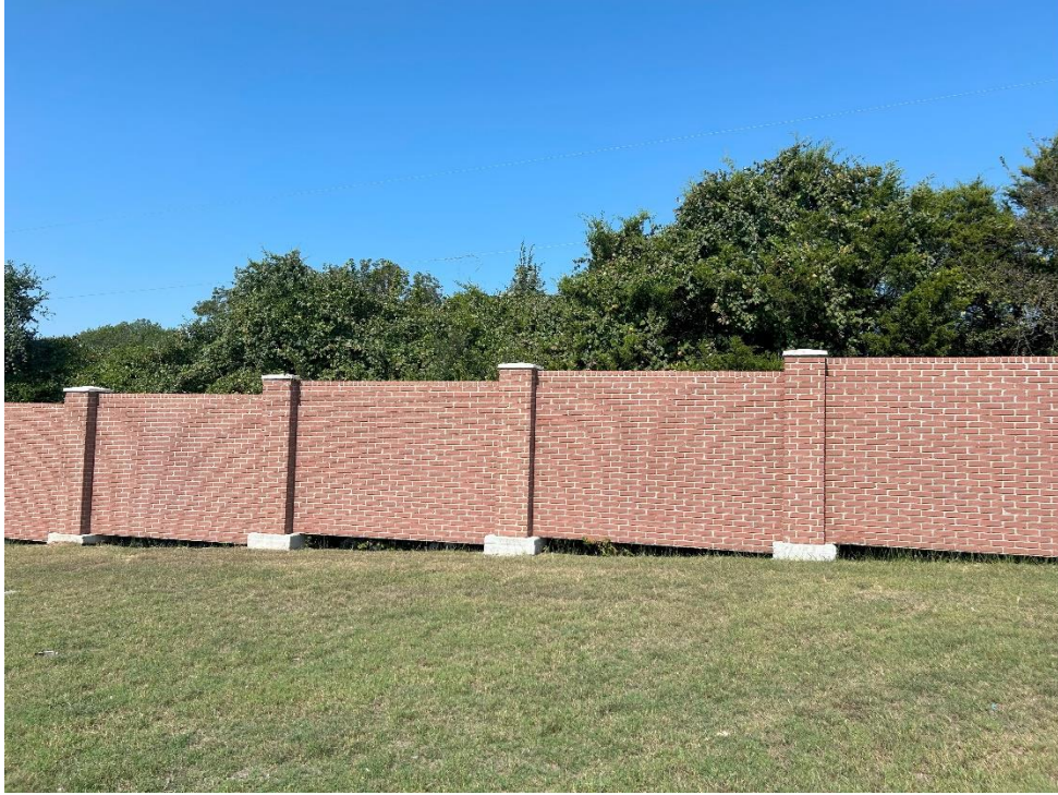
Precast wall at 215 W. Cartwright Rd
