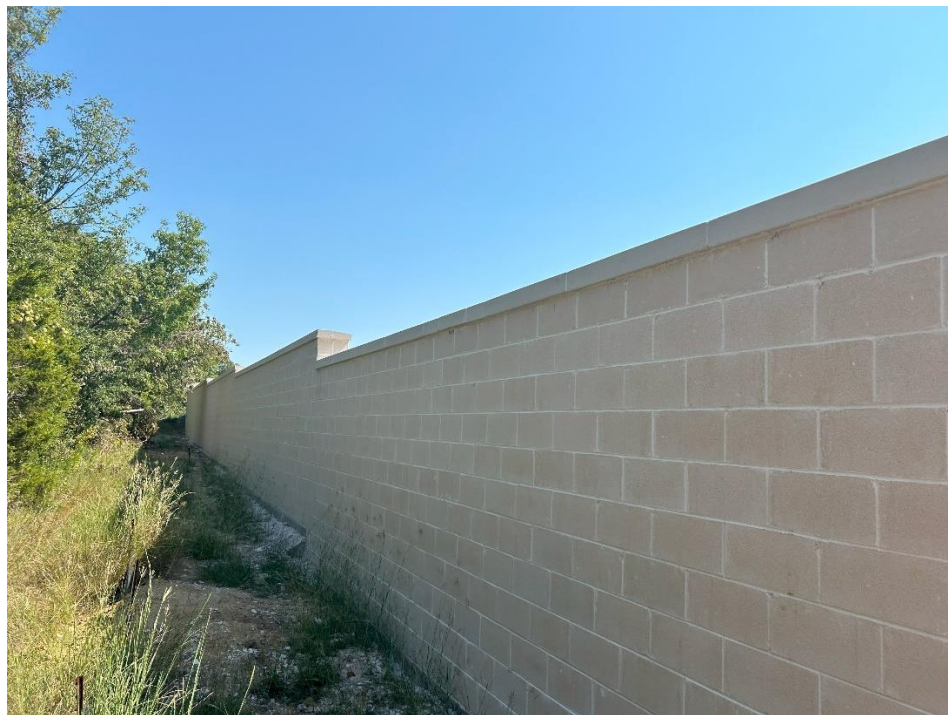
North side of the CMU wall
