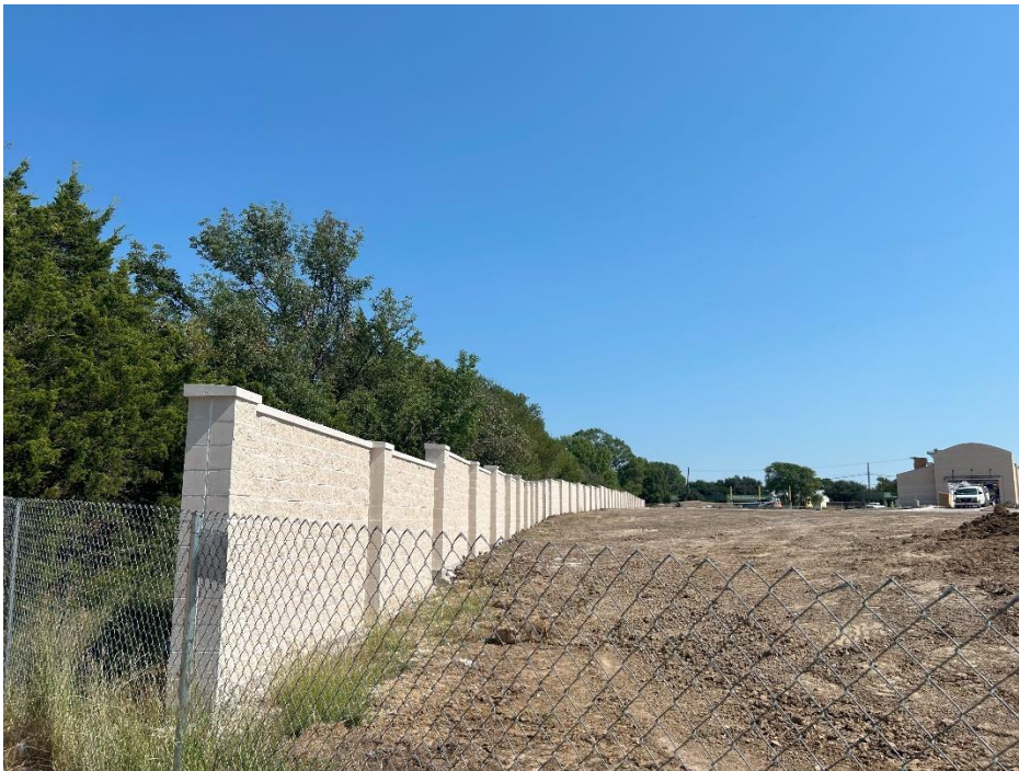
CMU wall from 215 W. Cartwright facing east
