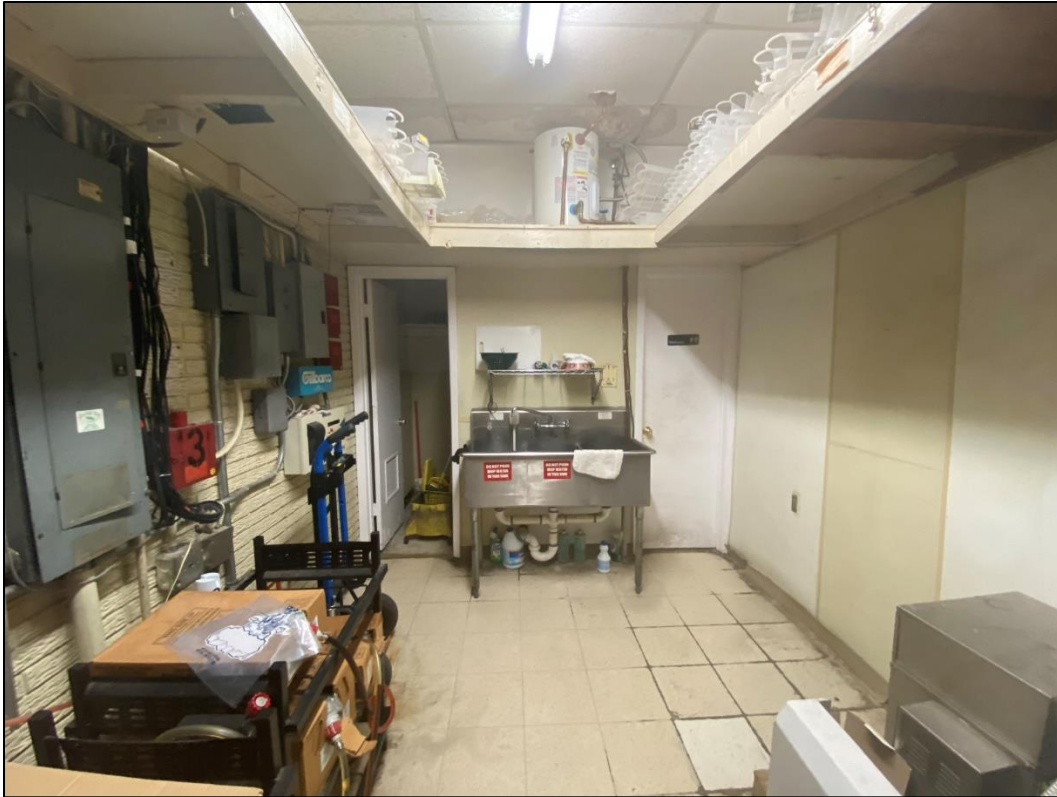
Storage area with restroom facility on the right (Unisex restroom).
