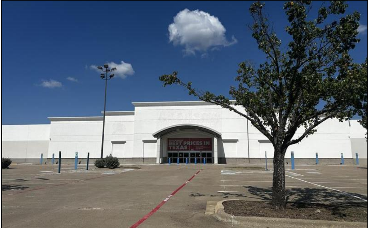
Subject property from parking lot, facing north.
