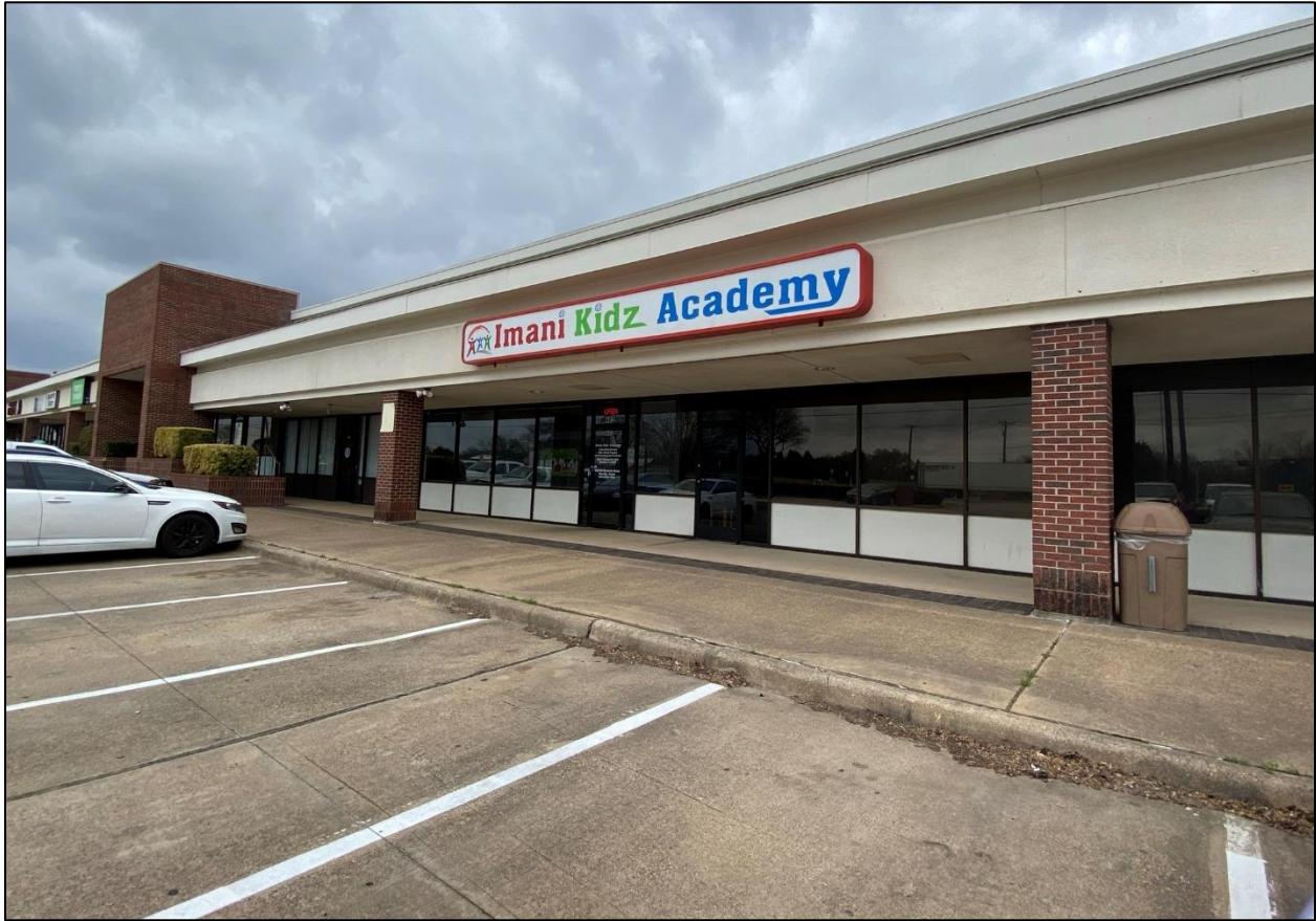
Existing child day care business in Suite 402, facing northwest.
