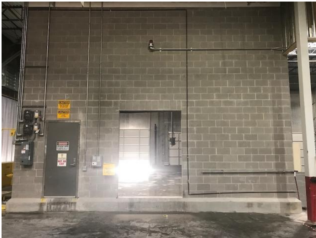
Explosion-proof enclosure for storing and mixing of chemicals.
