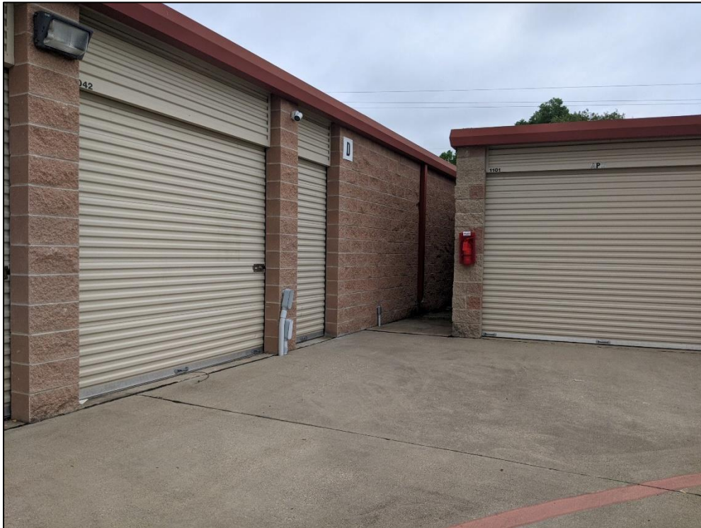
Separation (3 ft.) between Building C (right) and Building D (left)
